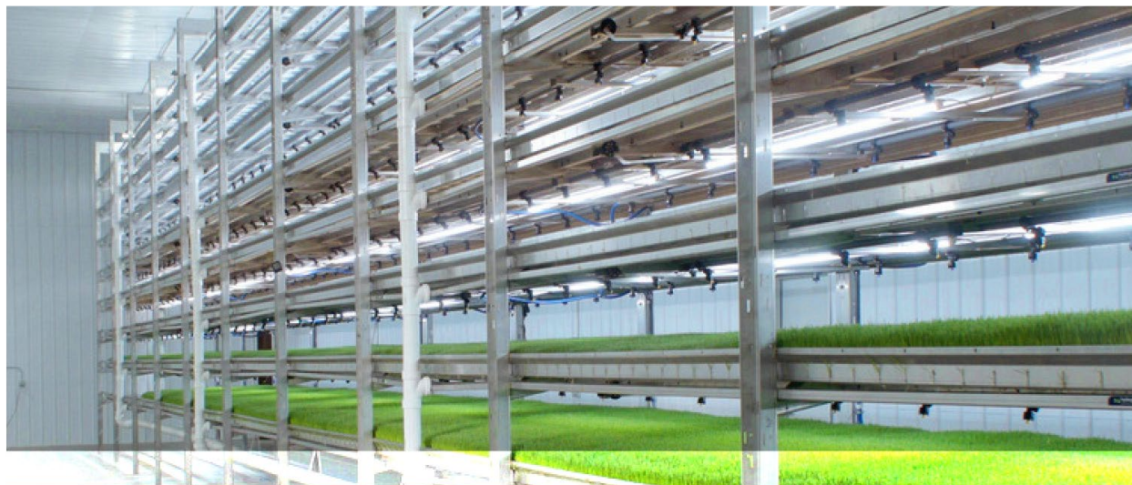
HYDROGREEN GROW SYSTEM
